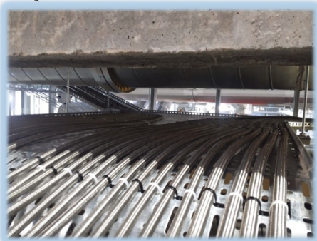
Virgin PTFE hoses installed on stainless steel trays throughout the manufacturing plant.
