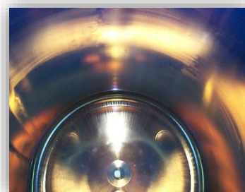
Figure 9 Rouge discolouration on the internal surfaces of a WFI storage
